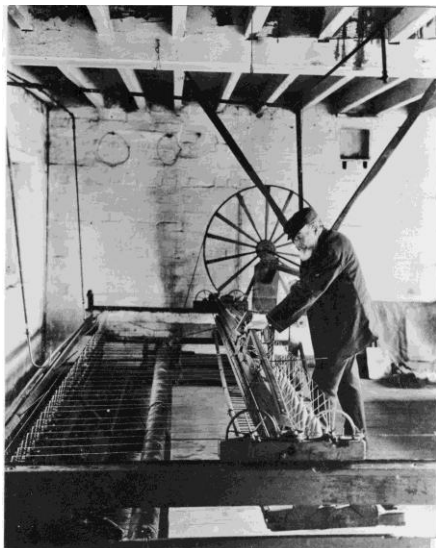
A spinning jenny being used in Palmer and Mackay's factory in Trowbridge
